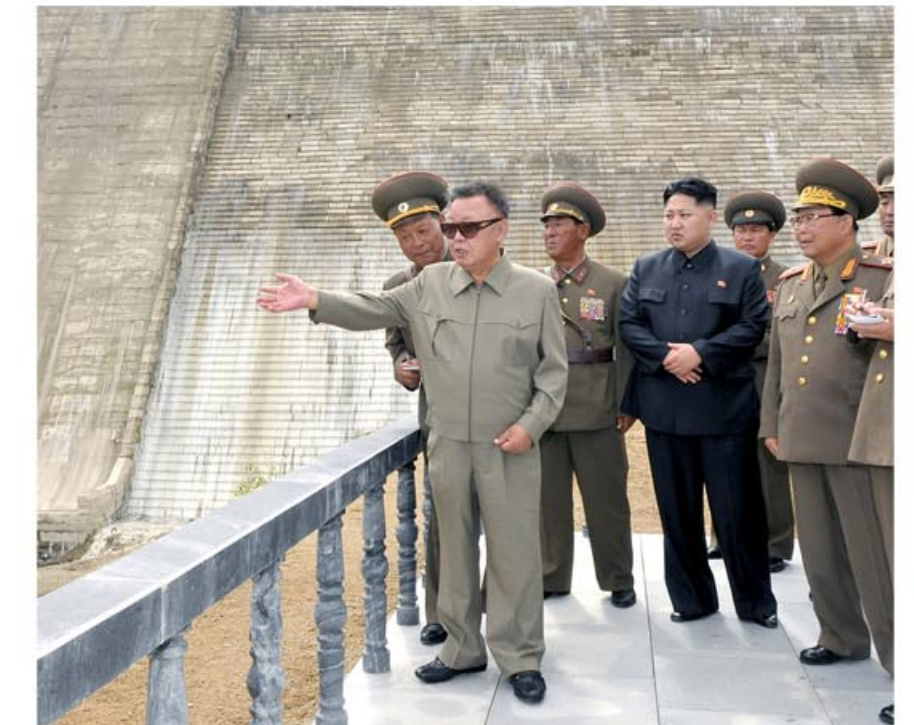
Kim Jong Il and Kim Jong Un give on-site guidance at the construction site of the Huichon Power Station (August 2011).
