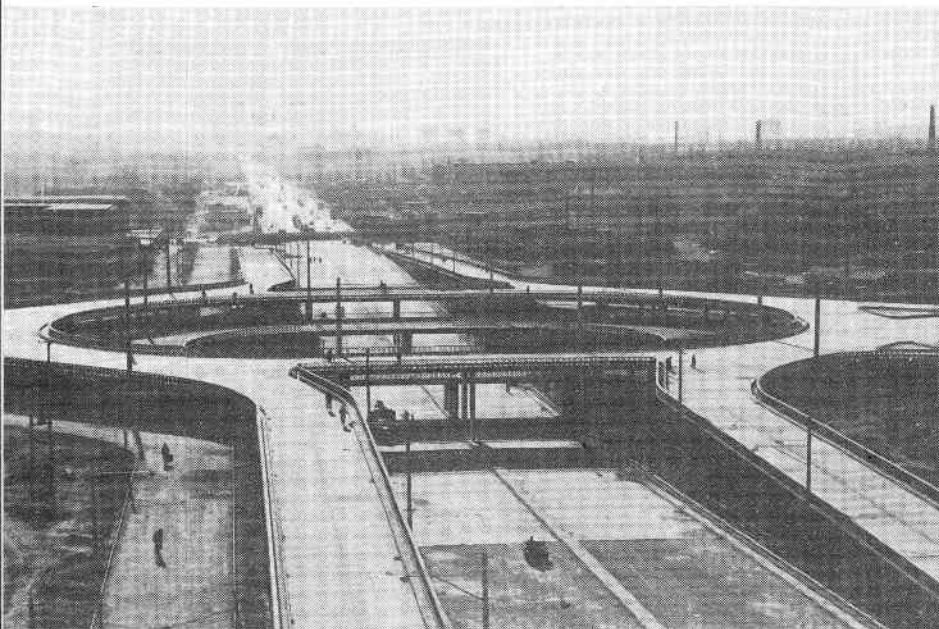
Three-level traffic circle at the former Xizhimen Gate.
